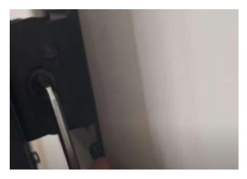
17 Any screws that are going into a stud use a 3/8 inch drill bit to create pilot holes in the stud.
