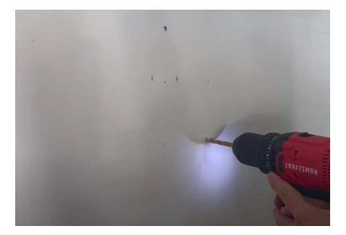
**11** For screws that are going into a stud use a 3/8 inch drill bit to create pilot holes in the stud.
