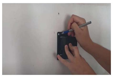
**10** For any screws that are not going into a stud, create a hole for the drywall anchors using a one-quarter inch drill bit
