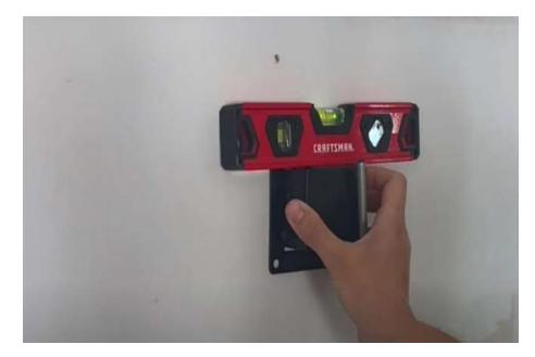
**9** Using the mount, hold it firmly in place and mark the location for the screw.
